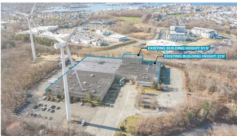
EXISTING SITE AERIAL
