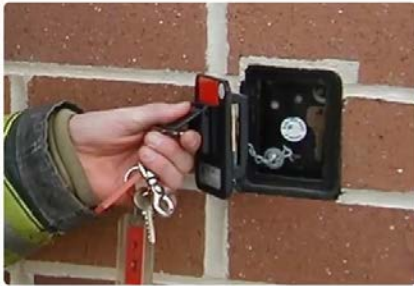
GFD HIGH-SECURITY EMERGENCY KNOXBOX INTERFACE
